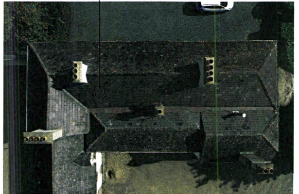
Section 5 Application Spring Farm, Kilquade, Co. Wicklow
